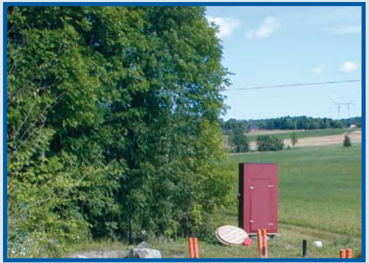
Photo 2 The pilot plant at Talby outside Stockholm. This plant treats sewage from Stockholm Vatten's office building at Bornsjön. The red shed contains sampling equipment used for taking daily and weekly samples.
