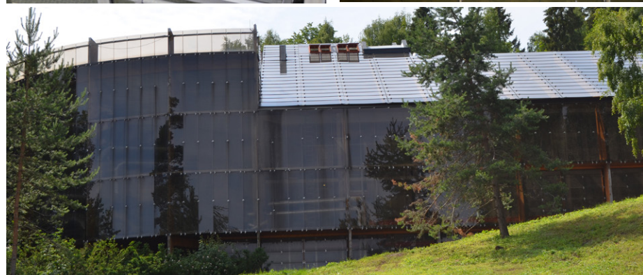
Elegant Veas building with all processes situated inside the mountain.
