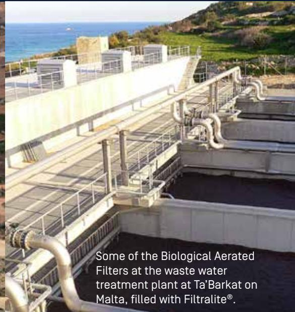
Some of the Biological Aerated Filters at the waste water treatment plant at Ta'Barkat on Malta, filled with Filtralite®.
