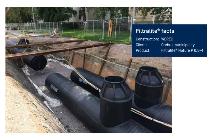
Bitumen, oil and rubber residues are separated in a pre-filter, consisting of an organic filter media. The pre-filter also contributes to metallic separation.
